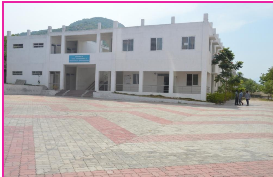
Mechanical & Civil Block
